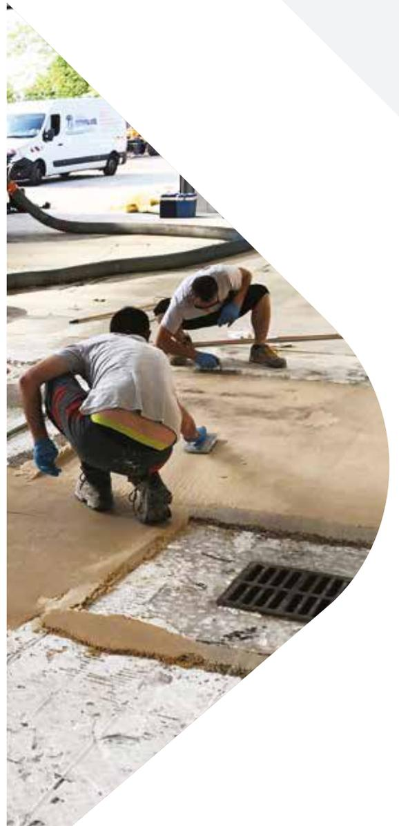
PRÉPARATION DES SUPPORTS, TRAITEMENT DES FISSURES ET RESTRUCTURATION AU MORTIER DE RÉSINE
