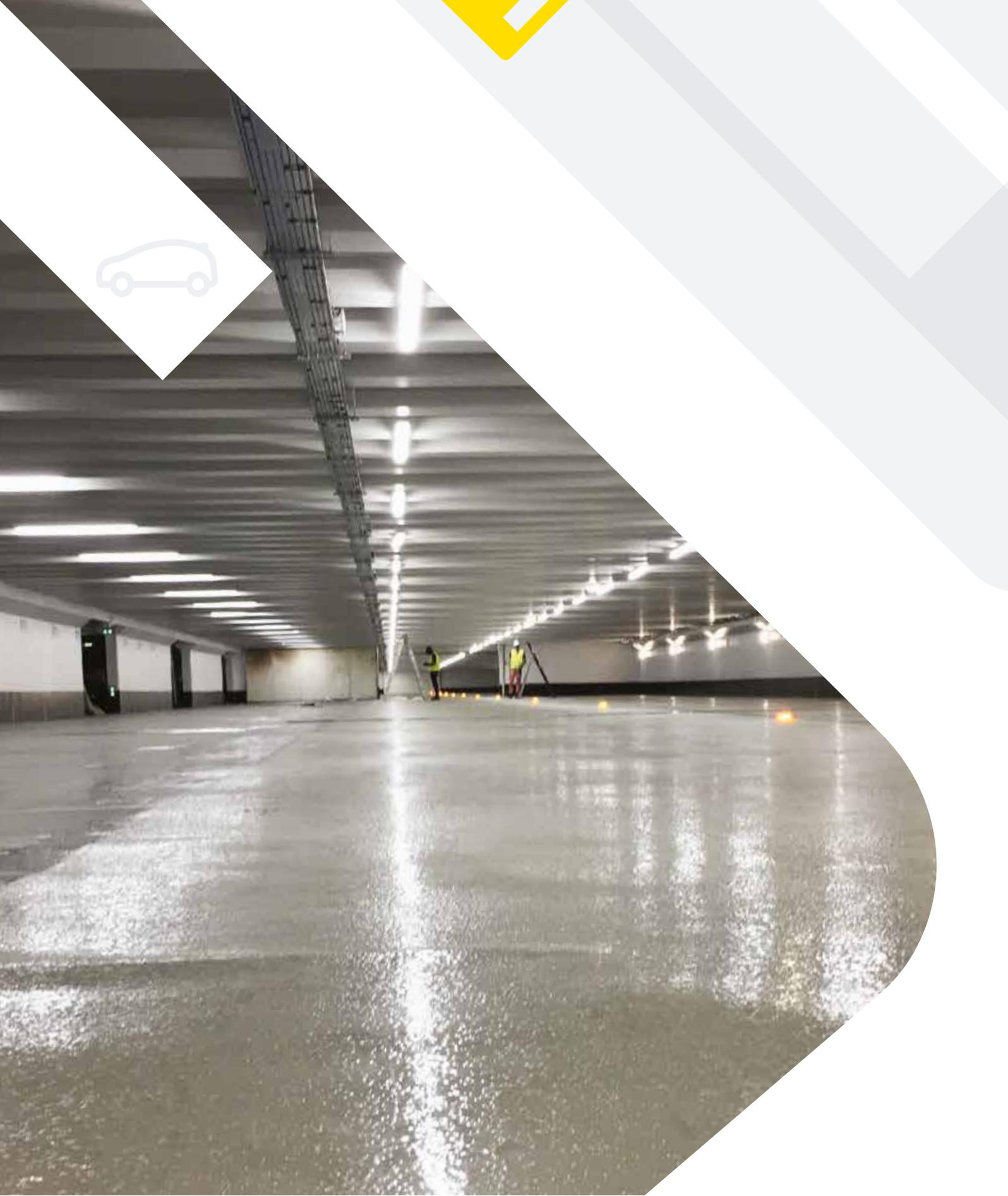
RÉALISATION D'UN SEMI-LISSE EN R.THANE 488 PERMETTANT L'ABSORPTION DES MICRO-VARIATIONS DIMENSIONNELLES DU SUPPORT
